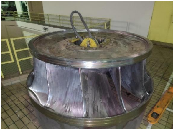
Figure 3 Marsyangdi Hydropower Turbine runner
